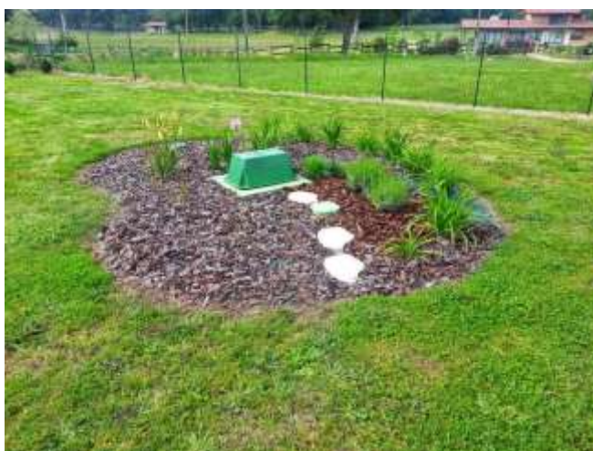
Micro-station Tricel Novo FR6/4000 installée
